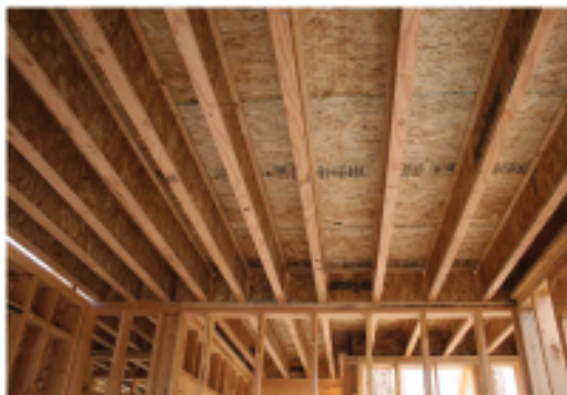
View of floor joists, beams and subfloor from below.
